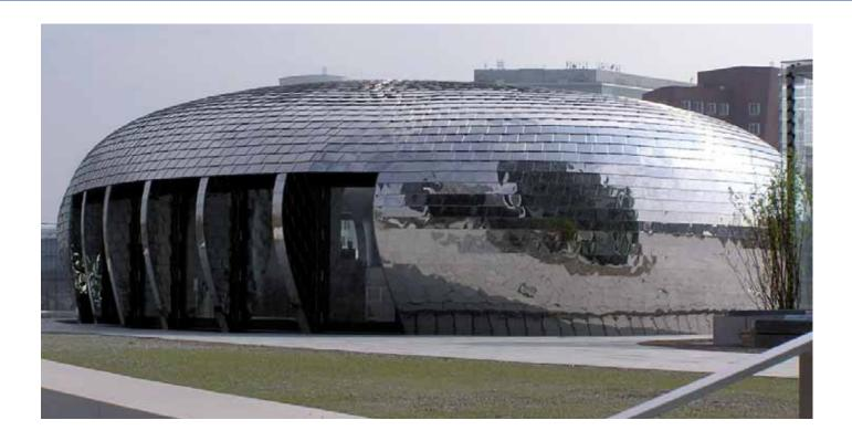
On account of its little expansion coefficient, stainless steel is an optimum material for roofs and fronts. It is not subject to cold brittleness. Backside-corrosion as a result of condensation water or entrapped moisture will no more occur.
