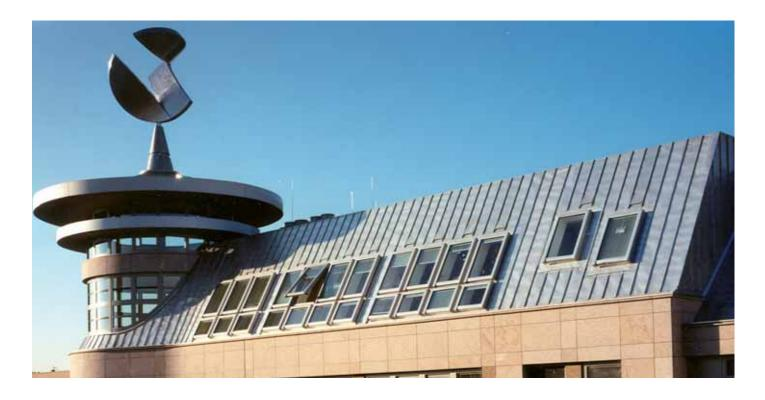
Tinned stainless steel (1.4509) is a rustproof, ferritic, 17 per cent chrome steel (magnetic) with 0,59 titanium content and an additional tin coating. For nearly 30 years it is used for roof coverings as well as roof drainage systems. Depending on its high corrosion resistance and a special applicability for restorations of landmarked buildings, it is very successful. Its matt-grey patina forms itself within a few years.
